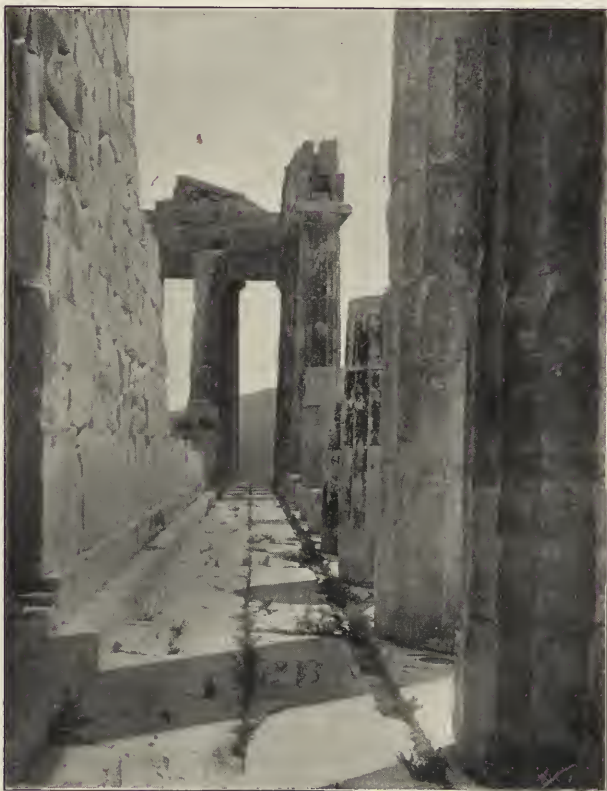
FIG. 48.—South Colonnade of Parthenon, showing inclination of Axes of the Columns.
